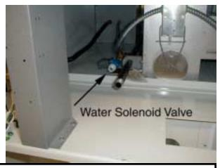
**IMPORTANT:** Flexible supply line/coupling *must be* used. Solenoid valve failure due to hard plumbing connections <u>WILL VOID WARRANTY</u>. <u>It is recommended</u> that a filter or strainer be installed in the water supply line.
