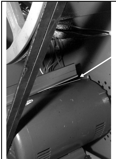
Figure 4: Close-up of Contractors Square Showing Degree of Motor Misalignment
